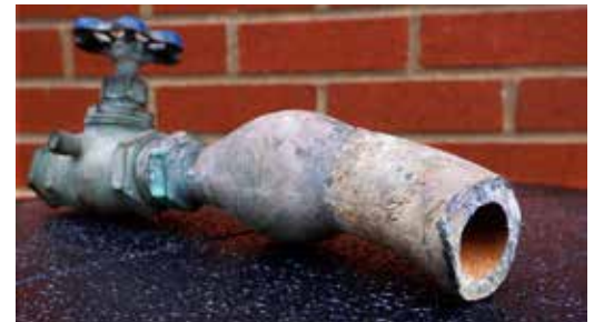
Image of a lead service line. Source: Associated Press.
